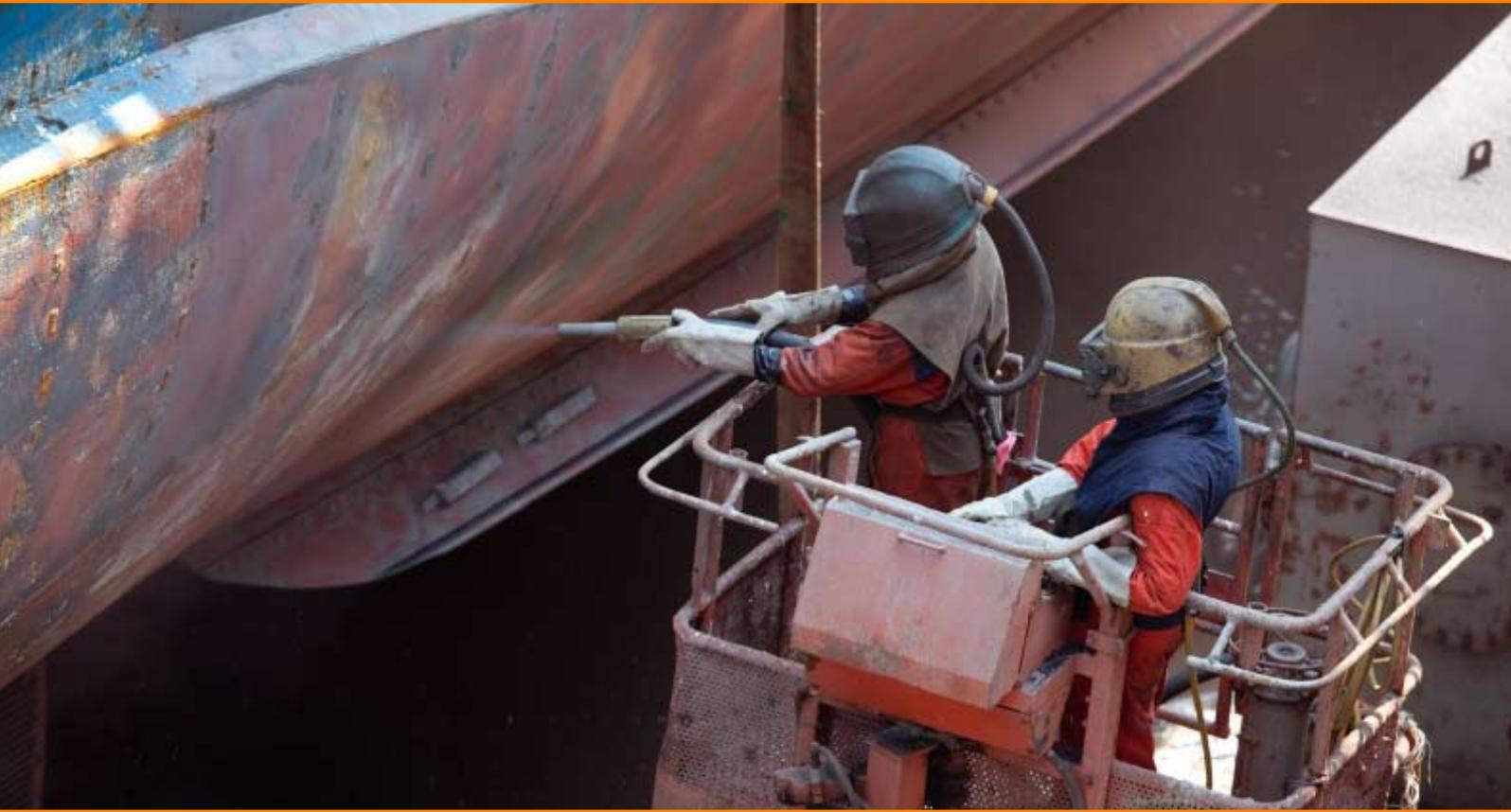
Airblast recognises the needs of the Anti Corrosion Industry and our abrasive blasting equipment offers all the features that the professional user requires. Our core range of open blasting pots all feature a well designed and proven single piece remote control & dead-man handle system and silencer ensuring reduced labour costs, high efficiency of abrasive utilisation, as well as operator safety.
